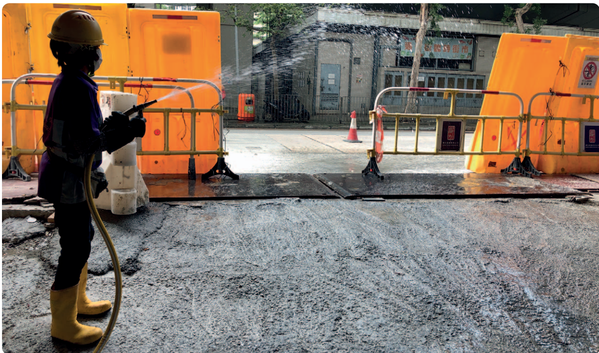
Regular water spraying at a construction site for dust suppression
